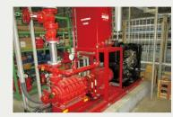
Electric motor and engine mechanism to drive fire hydrant pump
