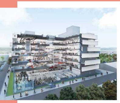
Japan Radio Co., Ltd. opened a new Advanced Technology Center in Nagano on December 8, 2014. The center has six aboveground floors and distinctive balconies on each floor. The building's total floor area is around 13,000 m<sup>2</sup>, but engineers also use the balconies to conduct research and test communications technology. Inside, each floor is open-plan with an atrium, and the layout is designed to make research more efficient and encourage cooperation between teams.
