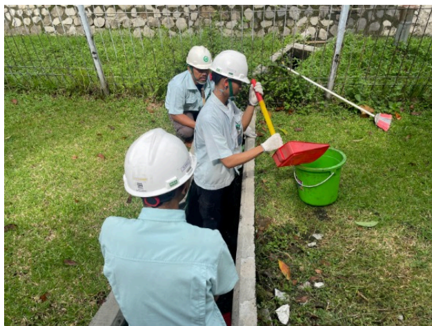
Training for handling leaks from outdoor drainage channels
