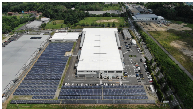
Solar power generation equipment for self-consumption
