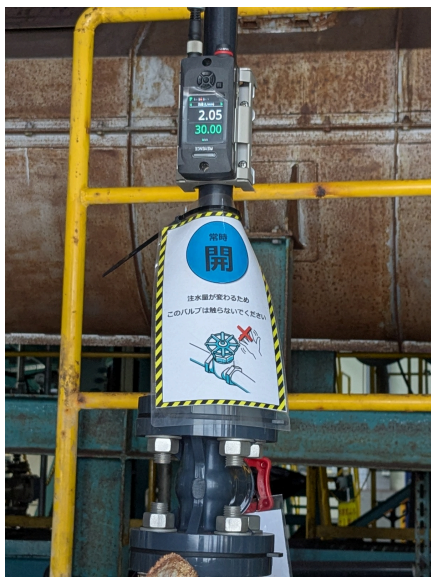
Flow meter added to supply pipe
