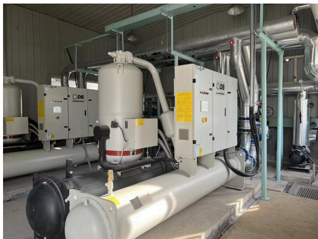
Energy-saving retrofitted air conditioning equipment
