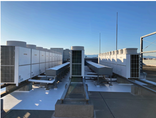
Air conditioning outdoor unit after heat shielding and insulation coating
