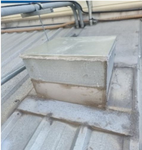
Removal of unnecessary ducts
