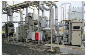
High-efficiency city gas-fired boiler
