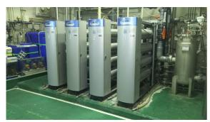
Wastewater reuse system (MRO) device
