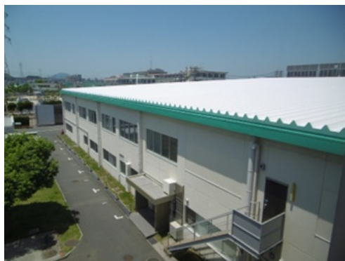
Painting with ceramic-based thermal barrier paint
