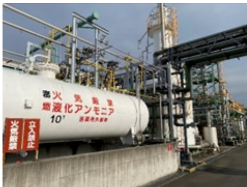
Liquid ammonia storage tank
