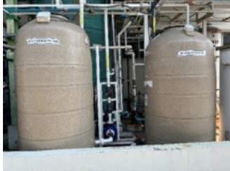
Dicing wastewater tank
