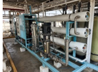
RO unit for producing pure water
