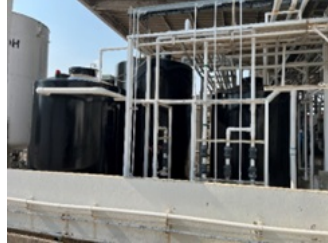
UF tank to contain wastewater
