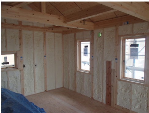
Residential insulation work using on-site spray foaming
