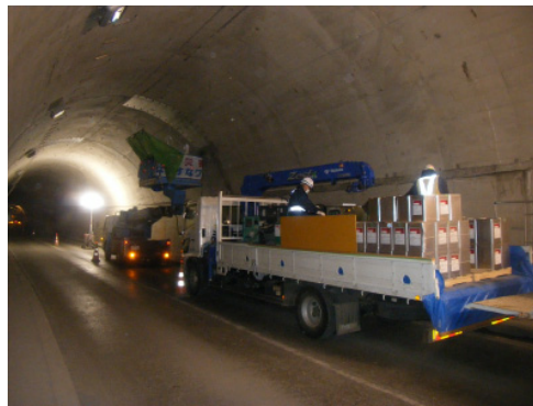
Repairing cavities behind a tunnel
