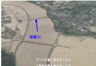
2020 Kuma River Damage
