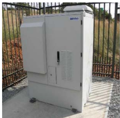
Fuel Cell for Emergency power supply
