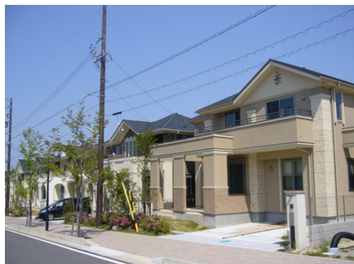
Redevelopment area in former Harisaki plant in Okazaki-shi, Aichi
