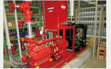
Electric motor and engine mechanism to drive fire hydrant pump
