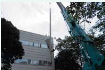
Tearing down the boiler smokestack
