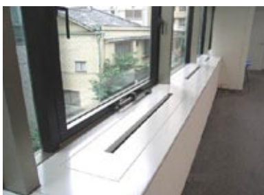
Air Barrier Fans (the vents below the windows) are sold by Nisshin Toa Inc.
