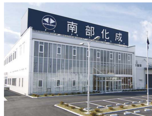
NANBU PLASTICS headquarters and techno center
