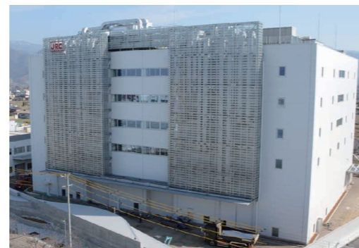
Japan Radio's production building
