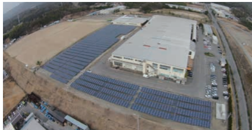
Nisshinbo Precision Instrument & Machinery Hiroshima Corporation's mega solar power facility
