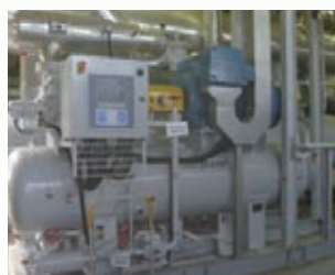
Ammonia cooling system
