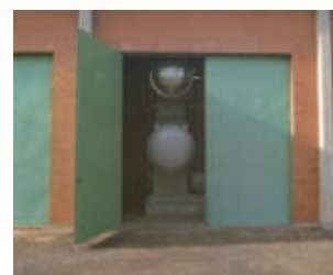
Ammonia cooling system in Factory No. 3
