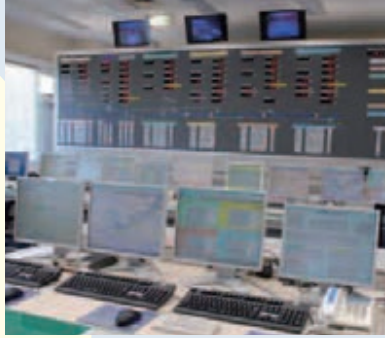
▲ Dam control system for Chubu Electric Power Co., Inc.
