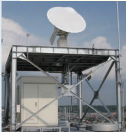
▲ Cutting edge weather radar installation (photo: National Research Institute for Earth Science and Disaster Prevention)
