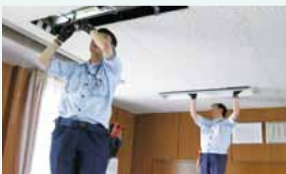
Work to replace fluorescent lamps with LED fluorescent tubes. Acting on its own initiative, Ueda Japan Radio replaced 100 fluorescent lamps in its office building.
