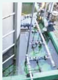
The broken valve
