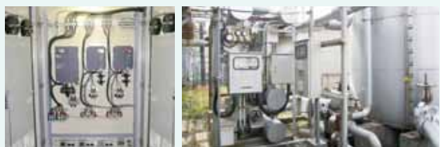
Conversion to mixed air conditioning inverters (Tatebayashi Plant)
