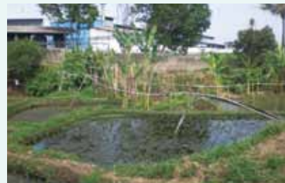
Water pipeline (off-site) The pipes are connected to cisterns scattered around outside the plant.
