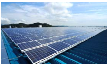
Nisshinbo Paper Products Inc. Shimada Plant Output: 250 kW Installation date: September 2010
