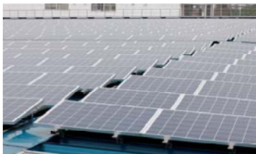
Nisshinbo Mechatronics Inc. Maii Machinery Plant Output: 250 kW Installation date: February 2010
