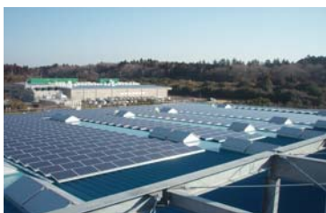
Nisshinbo Chemical Inc. Chiba Plant Output: 150 kW Installation date: February 2011
