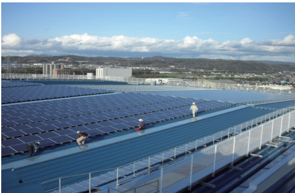
PV panels installed at the Mīai Machinery Plant of Nisshinbo Mechatronics Inc.
