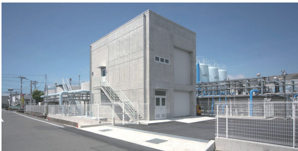
Waste water treatment facility (screw press located inside building)
