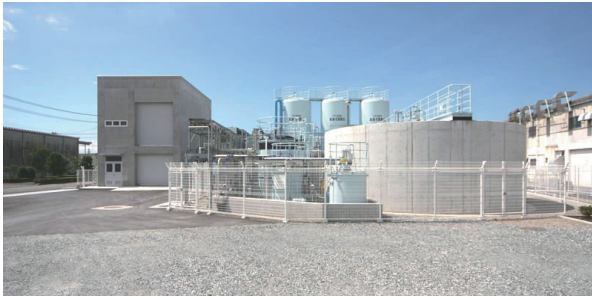
Supply and waste water treatment facilities (waste water side at far left, supply side at right)
