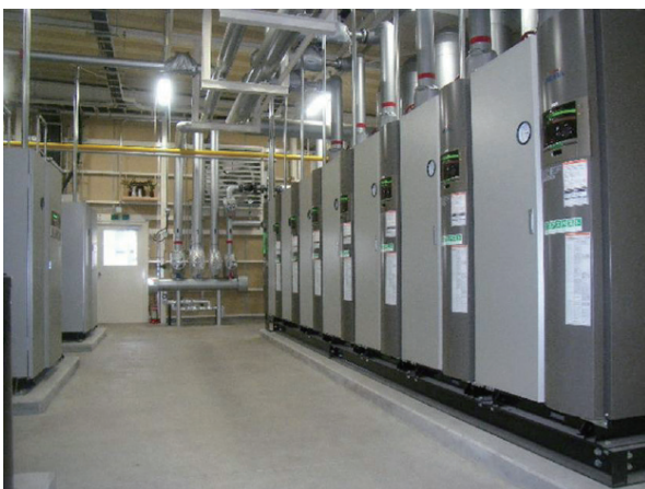
Town gas boilers
