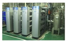
Wastewater reuse system equipment
